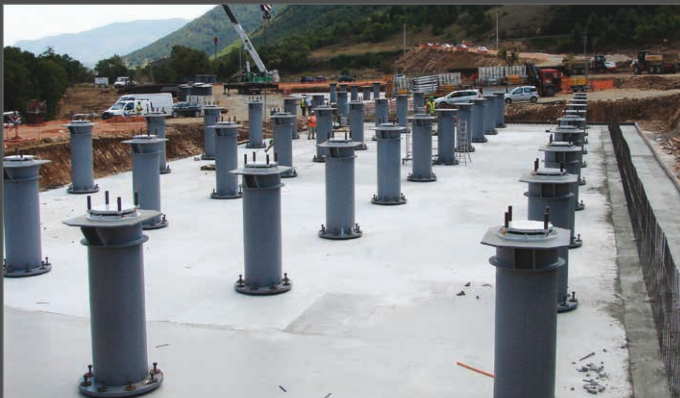
• L'AQUILA, ITALY - C.A.S.E. Project, installation of FIP-D
