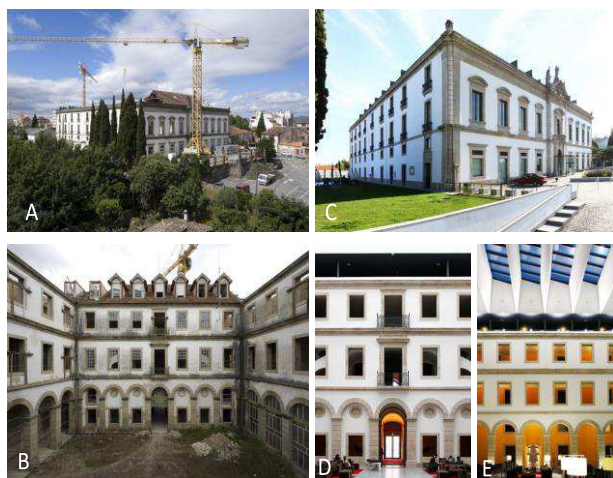
Figure 1. Overview of the Hospital's conversion works (A and B) and final appearance of the entire building of the Historic Hotel in 2009 (C, D and E). Photos from Santos [3].
