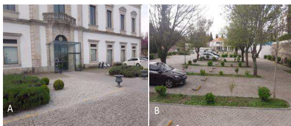
Figure 2. General view of the Hotel's main entrance (A) and the car park (B) before the implementation of the urban vineyard. Photos from authors.
