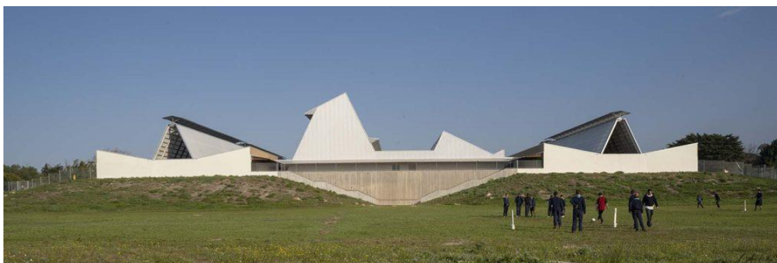
Figura 36 - Escola Cheré Botha, Cidade do Cabo, África do Sul (fonte: https://www.architectural-review.com/buildings/chere-botha-school-in-cape-town-south-africa-by-wolff-architects )
