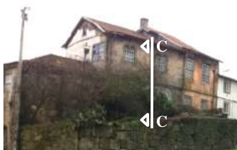
a) Fachada principal
