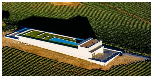
Figura 13 – Adega Mayor – cobertura verde
