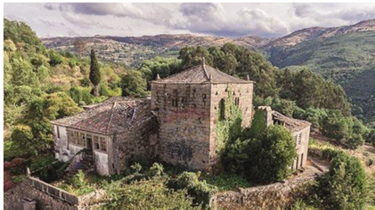
Figure 1. House at Torre da Lagariça property current state.
